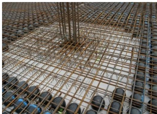
1: Bubble Deck Slab
