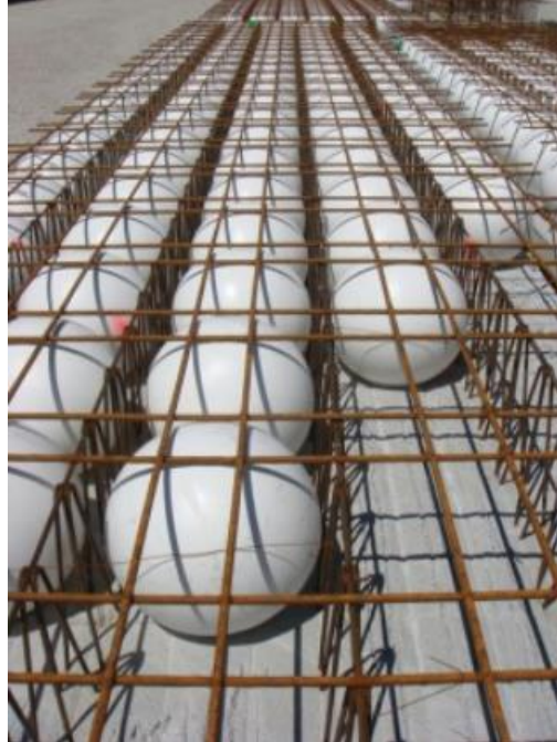
Bubbles used in the Bubble Deck slab.
